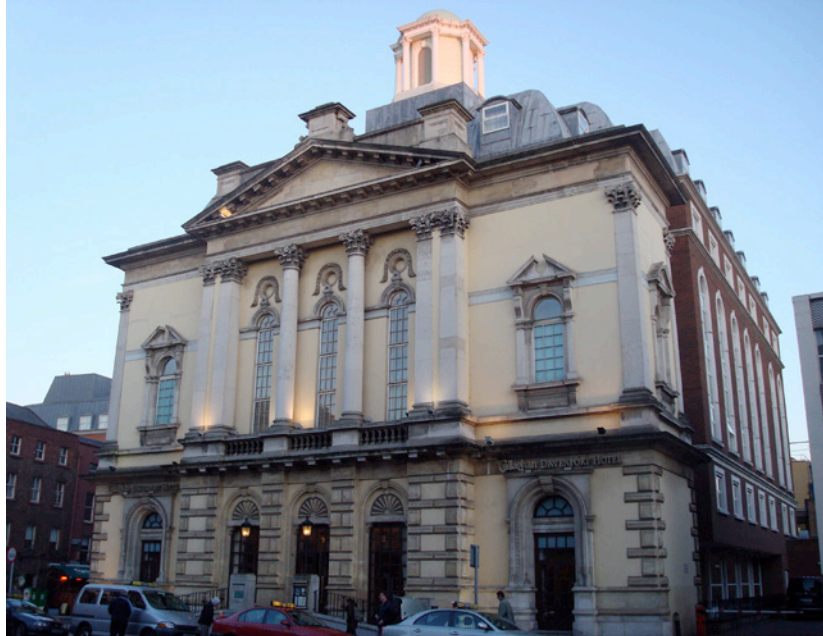
Merrion Hall, Dublin
